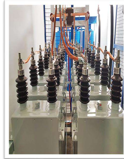
Unbalanced detection scheme capacitor
